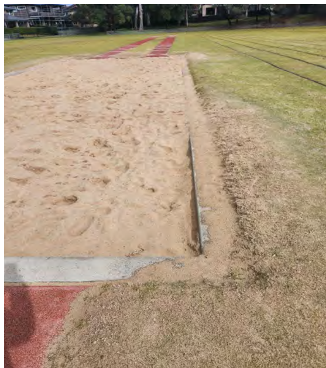
Image 5 – photo of exposed edging around the existing long jump pits
